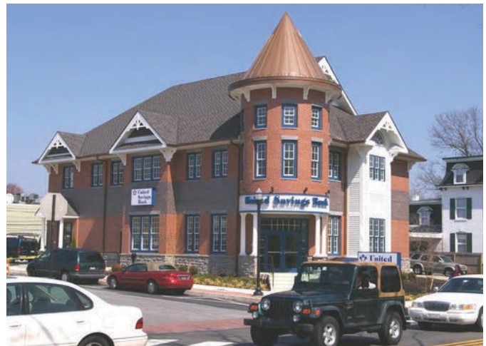
Articulated Facade with Vertical Bays, and Articulated Roof, United Savings Bank, Media, PA
