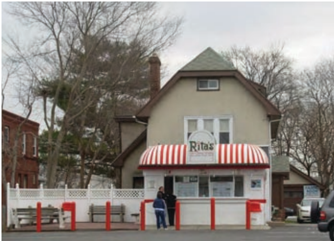
Apartment Above Water Ice Stand, Eagle Road
