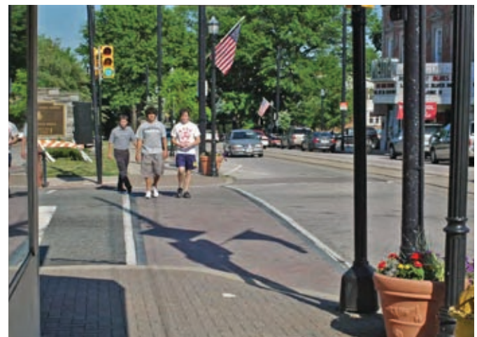
Best Practices example of Raised Unit Paver Crosswalk at Grade, Media, PA
