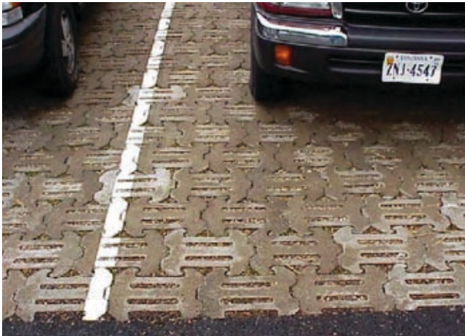
Unit Pavers as Porous Pavement
