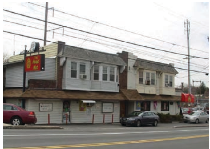
Buildings Located Close to Sidewalks along Haverford Road
