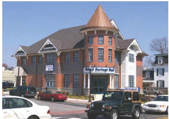
Articulated Facade with Vertical Bays, and Articulated Roof, United Savings Bank, Media, PA
