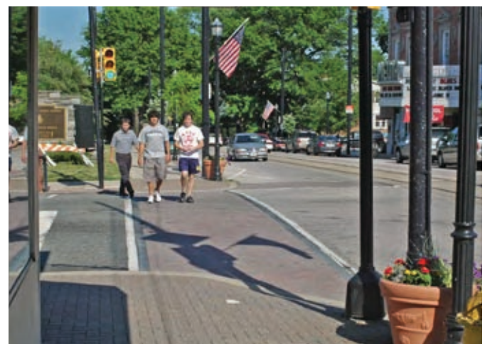
Best Practices example of Raised Unit Paver Crosswalk at Grade, Media, PA
