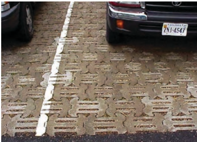
Unit Pavers as Porous Pavement
