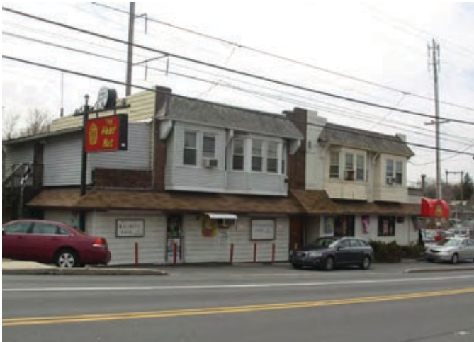
Apartments Above Commercial, Haverford Road
