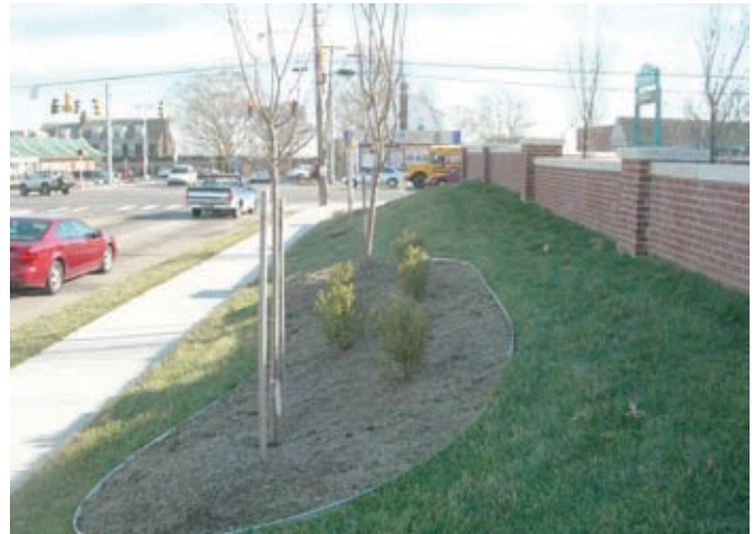
Example of Best Practice for Street Wall of new Wawa in Claymont, Delaware, Buffering Off-street Parking Lot.
