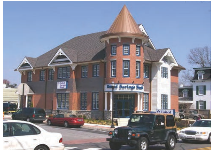
Articulated Facade with Vertical Bays, and Articulated Roof, United Savings Bank, Media, PA
