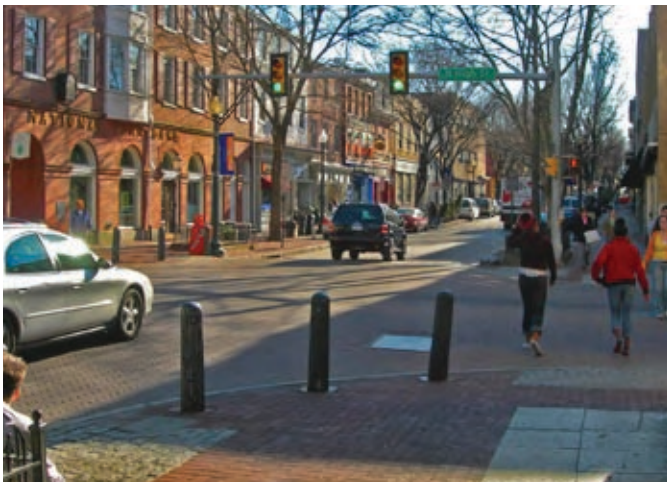
Best Practices example of Speed Table Crosswalk, West Chester, PA
