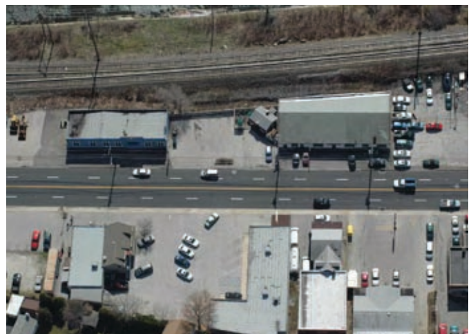
Wide Curb Cut Along Haverford Road Increases Vehicular and Pedestrian Conflicts
