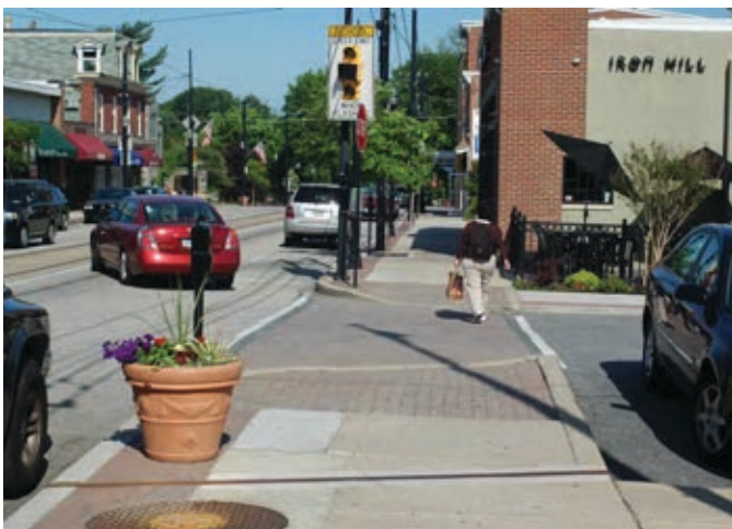
Sidewalks with Small Curb Cuts Reduce Pedestrian and Vehicular Conflicts in Media, PA
