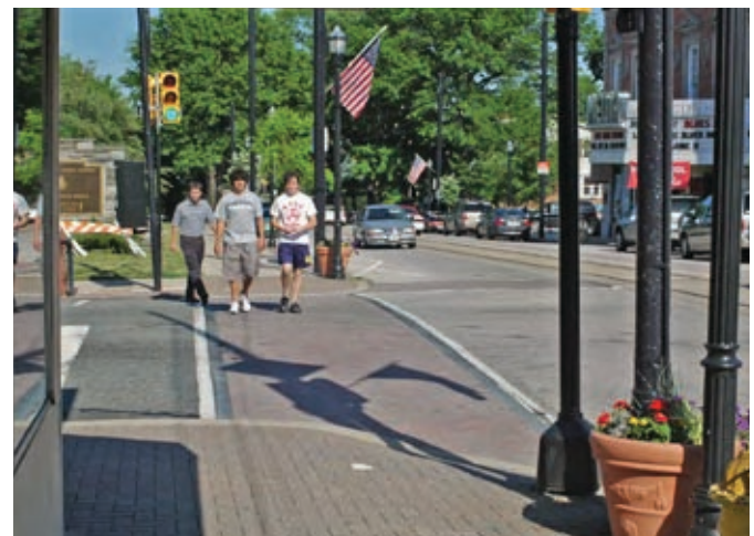
Best Practices example of Raised Unit Paver Crosswalk at Grade, Media, PA
