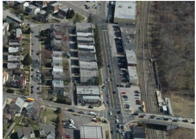
Buildings Grouped Close Together, Haverford Road
