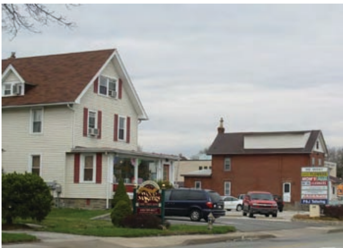
Enclosed Porch Reduces Building Permeability Along Eagle Road
